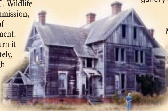
The main Keepers' house in 1979 before restoration.
