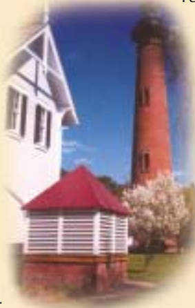
The cistern after restoration.
